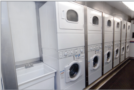
View of the sink, washers, and dryers
